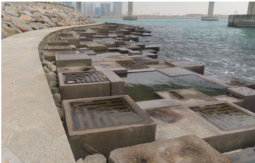
General View of Rocky Eco-shoreline
